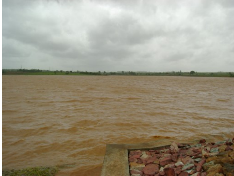
Plate1: A panoramic view of completely filled Narendra tank
