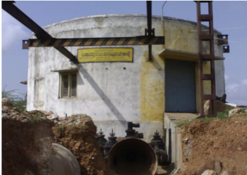
Plate3: Ekhaspur lift irrigation scheme suffering from inadequate power supply
