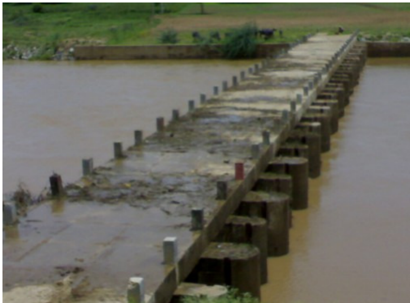
Plate6: A view of completely filled Lingadahalli barrage
