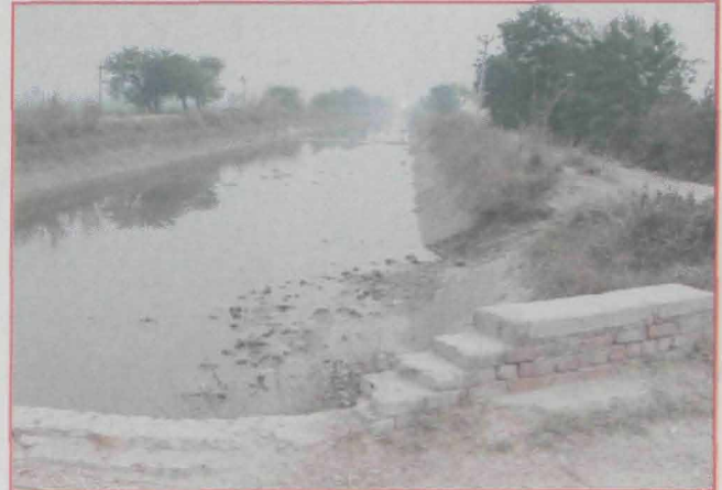
Figure 19. Sunder canal branch
