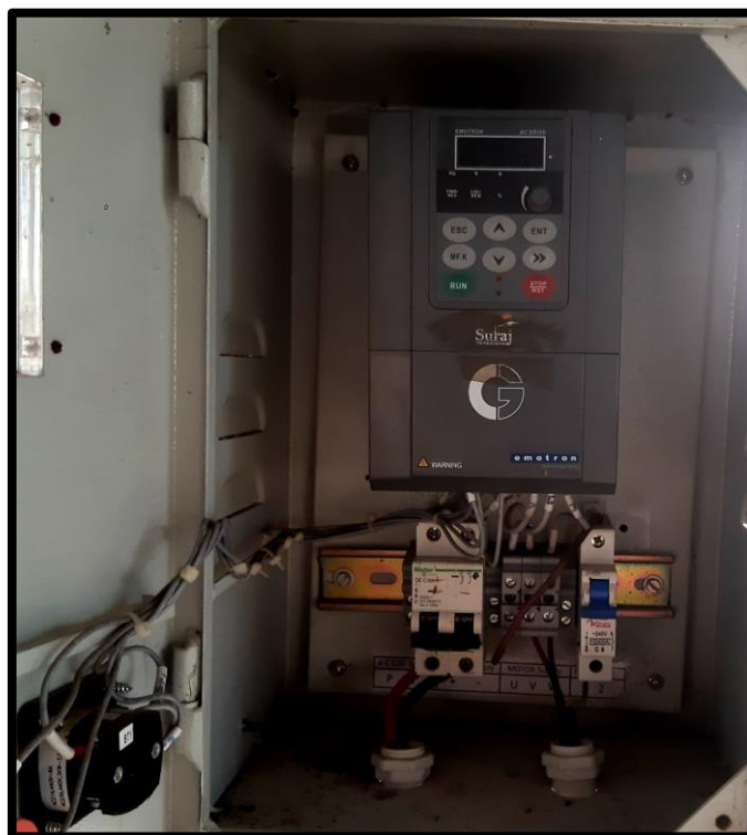
Plate 3.3 : Variable Frequency Drive
