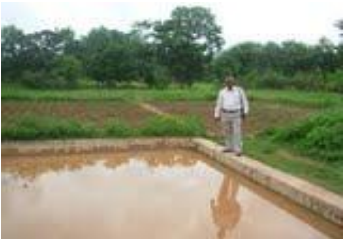
Fig 4.41 Water harvesting pond with water
