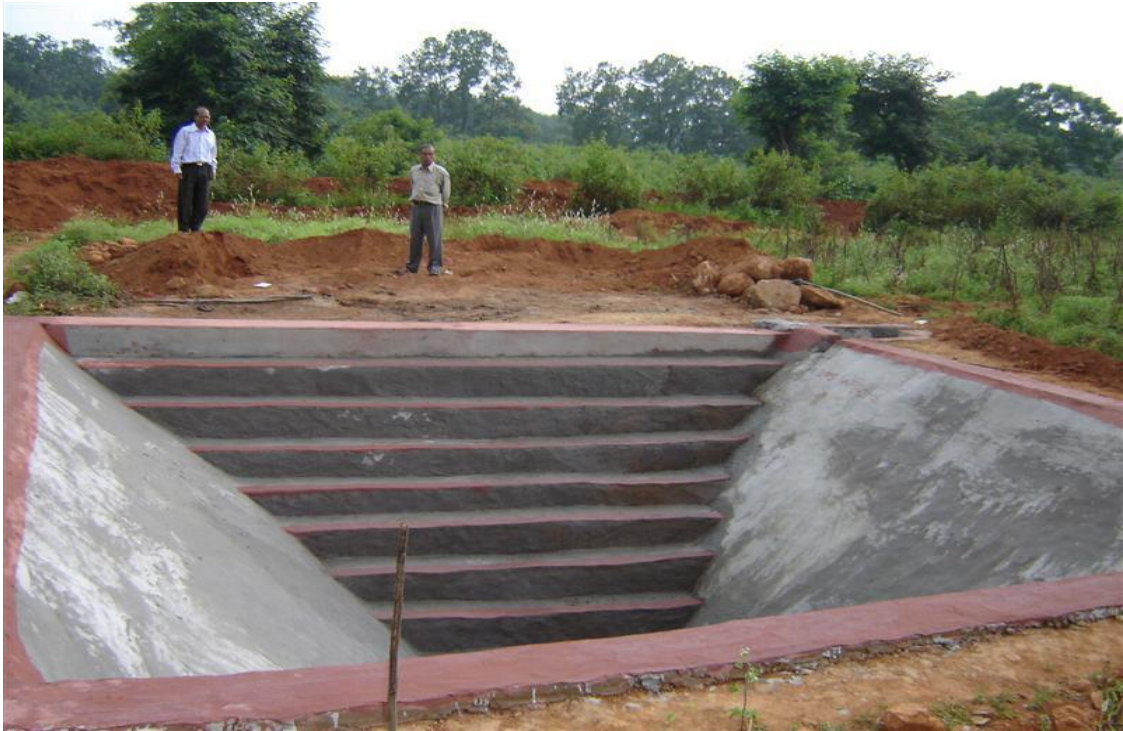
Fig 3.5 On farm reservoir with soil cement (6:1) plaster lining
