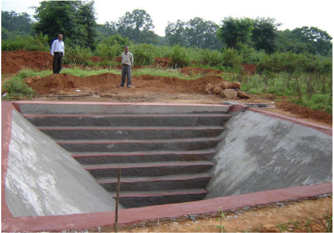
Fig.4.40 Water harvesting pond without water
