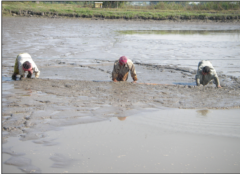
Plate 70: Dewatering using iron pipe
