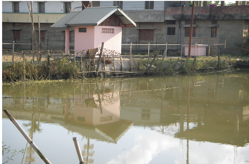
Plate 72: Bamboo poles to prevent from erosion
