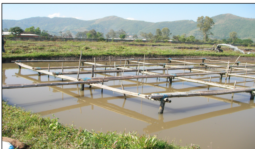
Plate 69: Wooden frame for fixing Hapa
