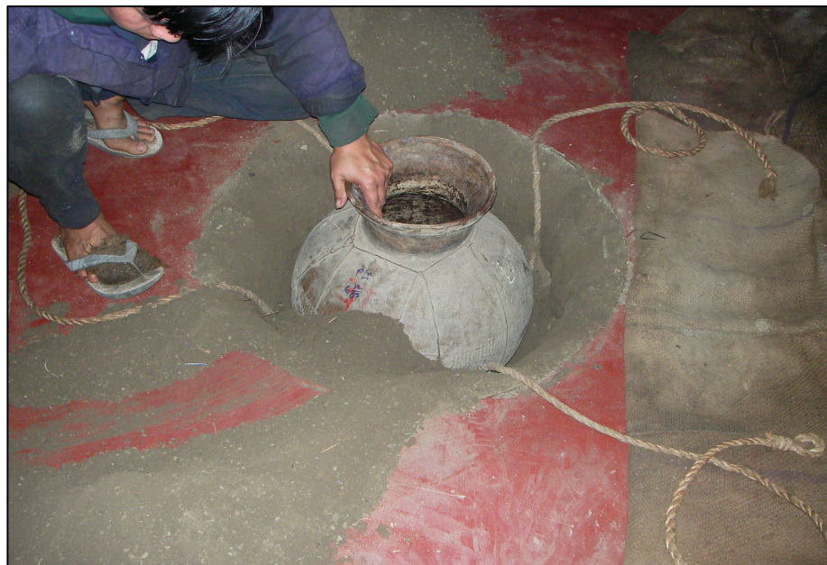
Plate 38: Fixing the earthen pot inside the pit
