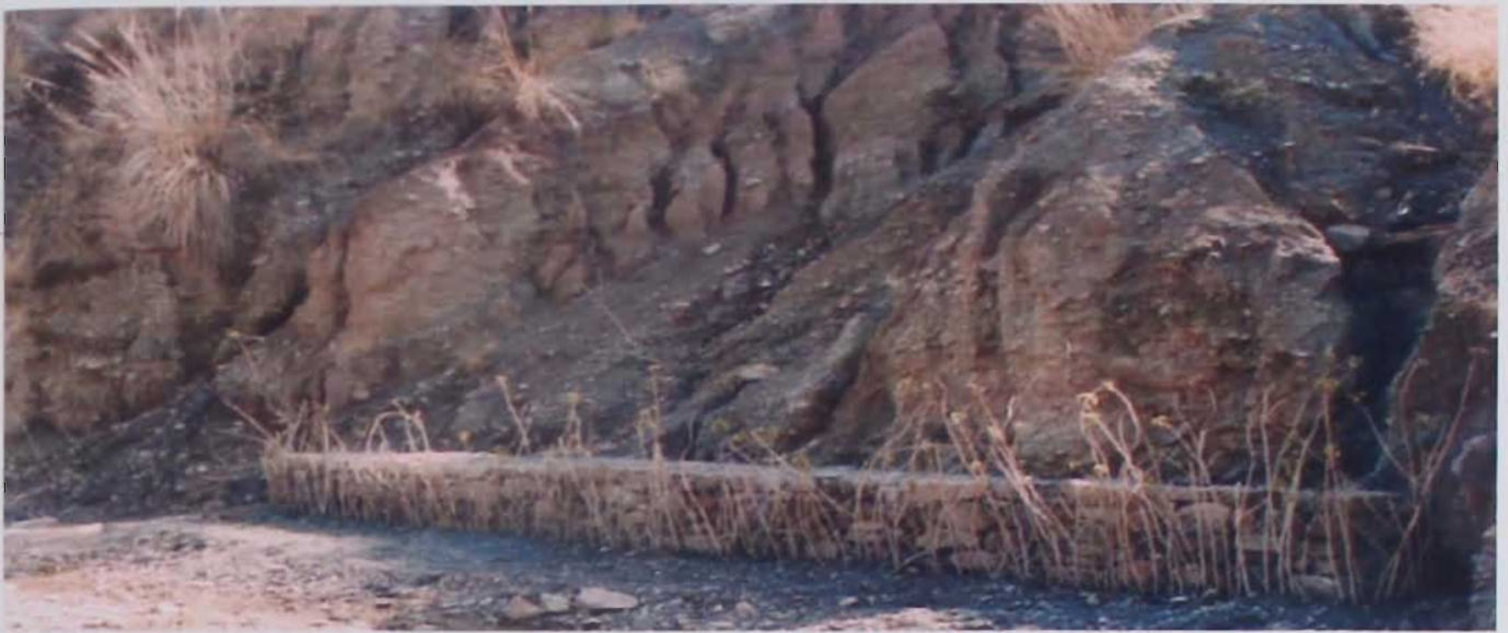
A. Mechanical measure - retaining wall (Gabion wall)
