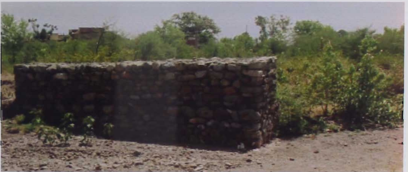
B. Mechanical measure - Attracting type spur
