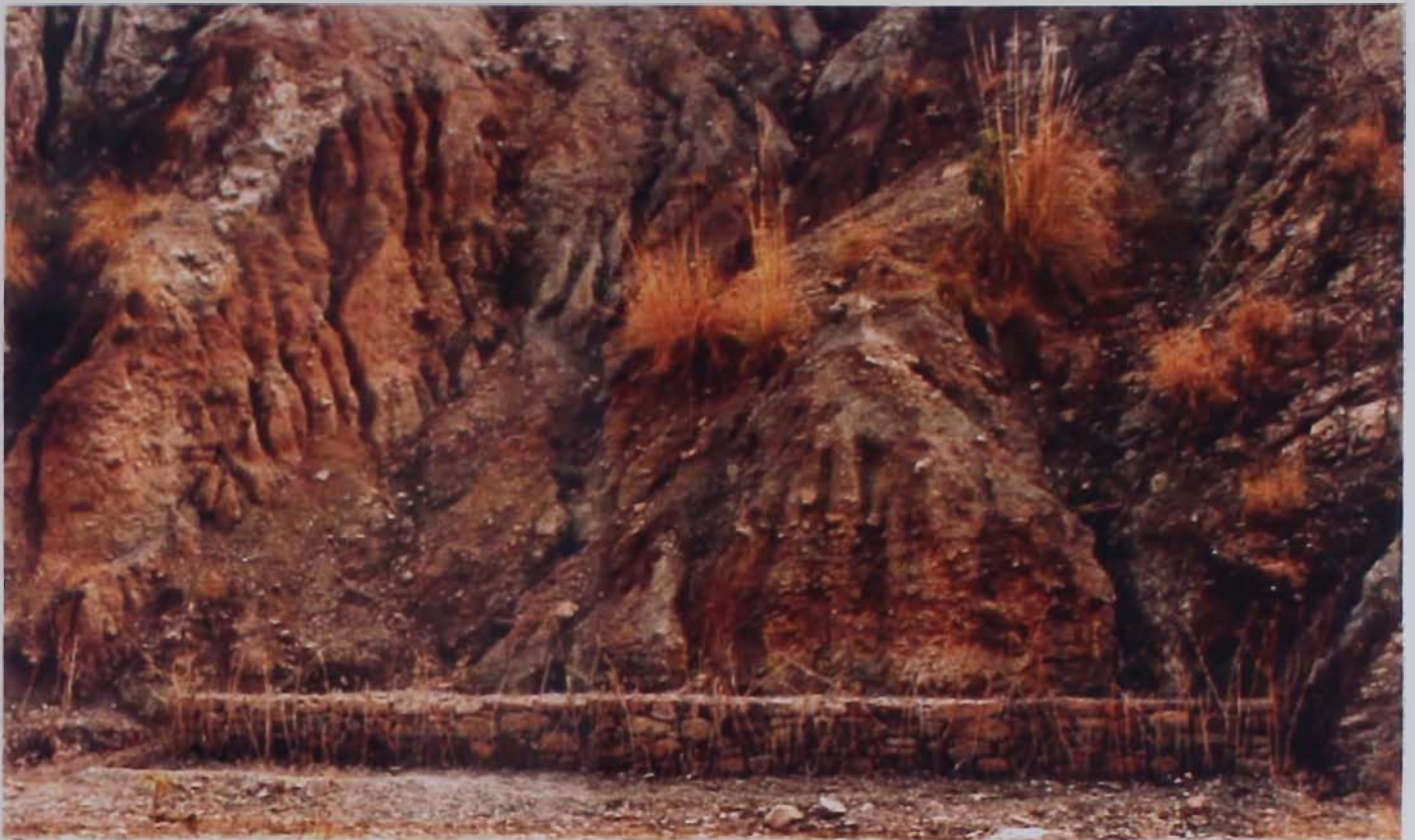
A. Retaining wall constructed in 2004
