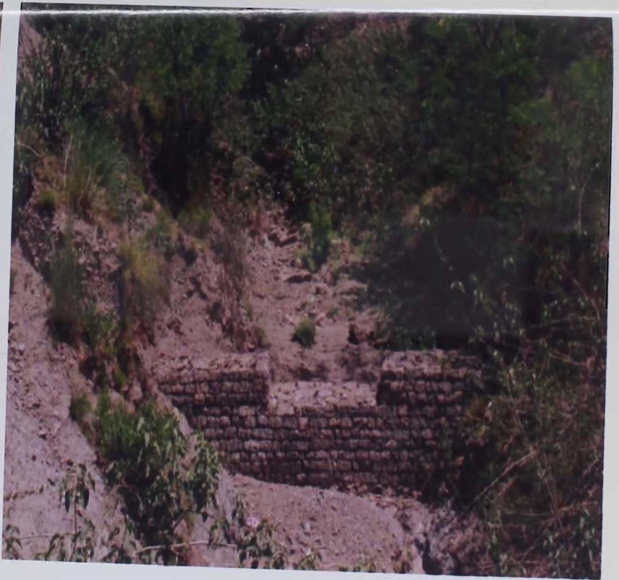
B. Gabion Check dam
