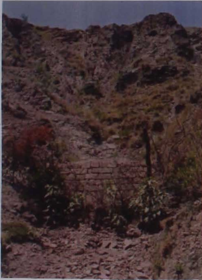
A. Mechanical+vegetative measures in upper part of catchment (Loose boulder check dam reinforced with Ipomoea cuttings)
