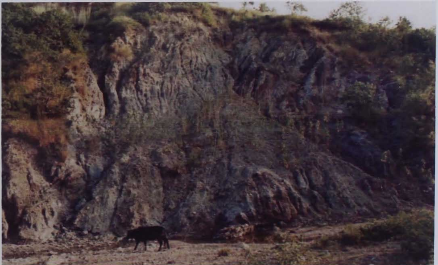
B. Retaining wall buried under landslide in 2006
