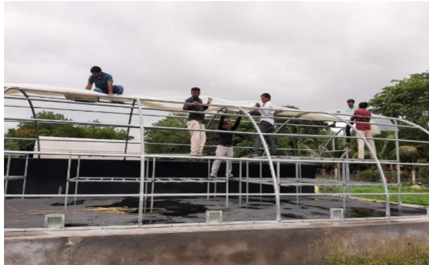
Plate 3.2 (a) Inside frame structure of solar tunnel dryer
