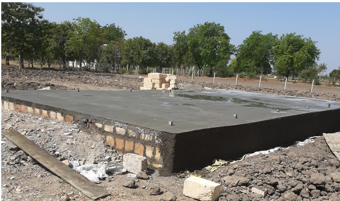
Plate 3.1 Construction, insulation and plastering of RCC platform of solar tunnel dryer
