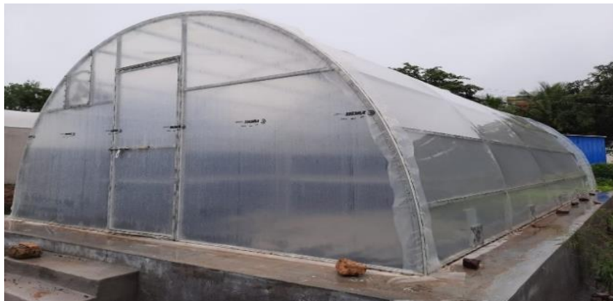
Plate 3.2 (b) Solar tunnel dryer covered with 200 \mu UV stabilized polyethylene sheet
