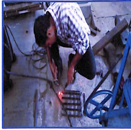
b) Fabrication of compartmental unit
