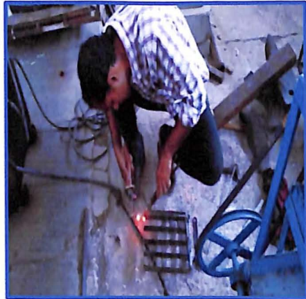
b) Fabrication of compartmental unit
