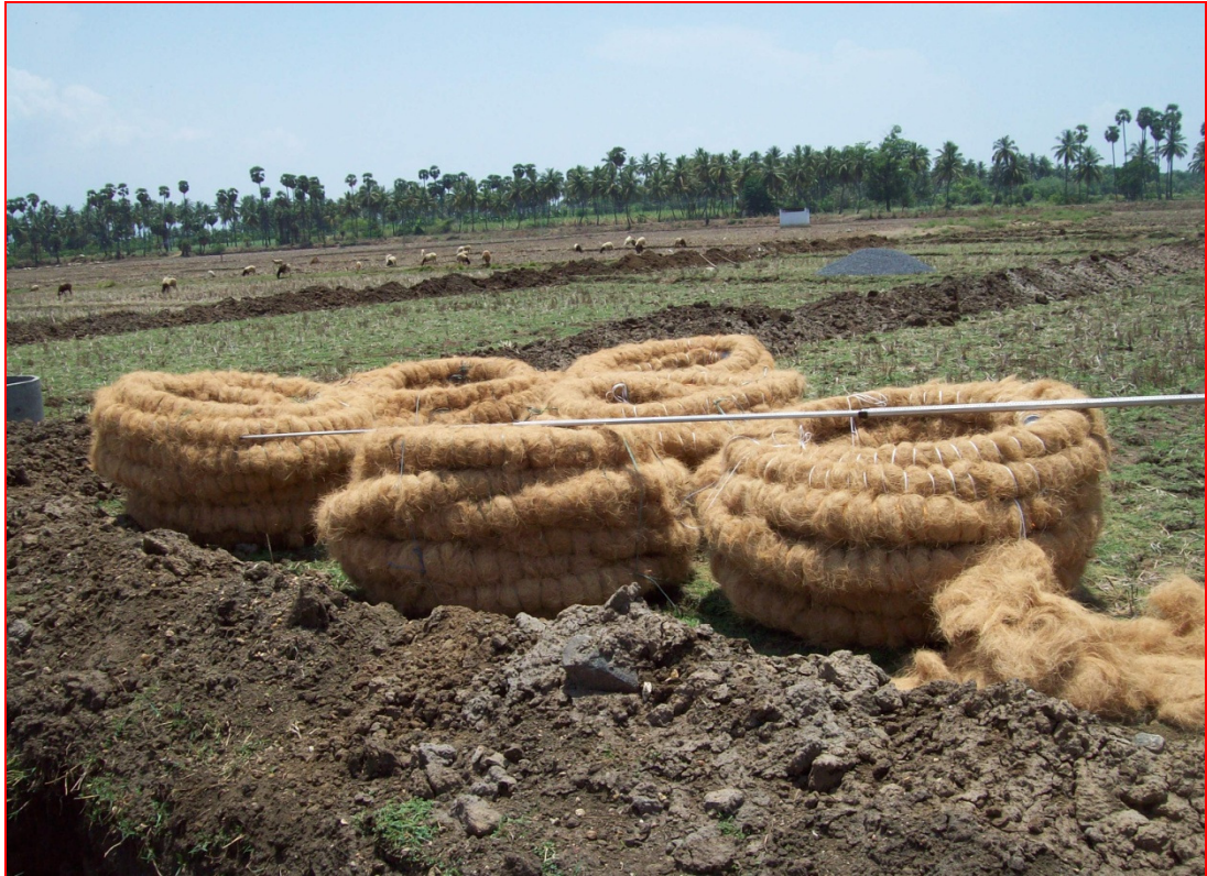
Plate 3.7 Coconut coir wrapped drain pipes of required length
