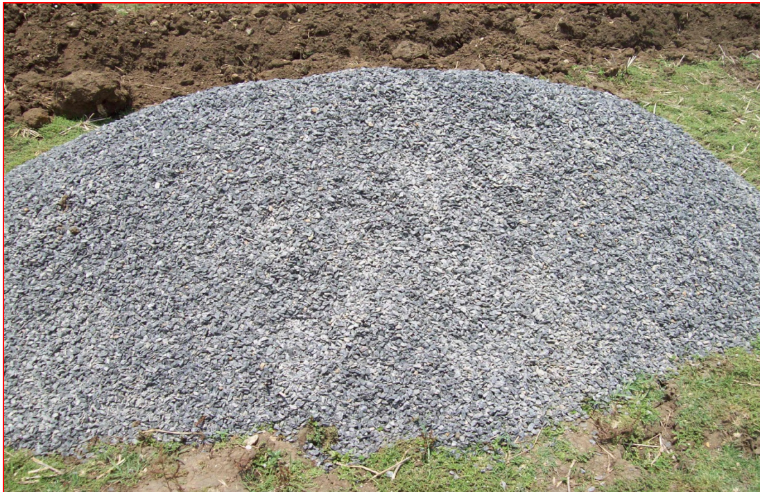
Plate 3.8 Zero chips for bedding material kept ready for placement
