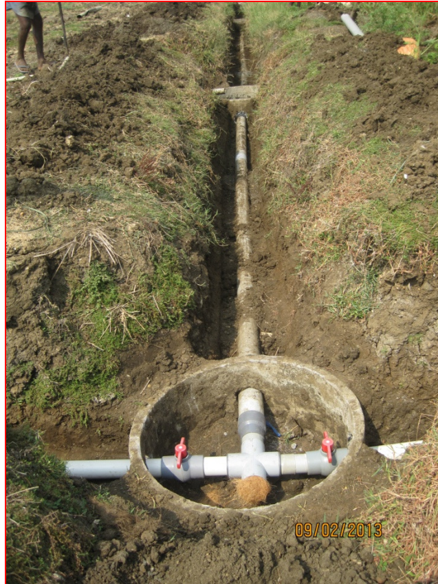
Plate 3.13 Interconnection of collector and laterals for subirrigation
