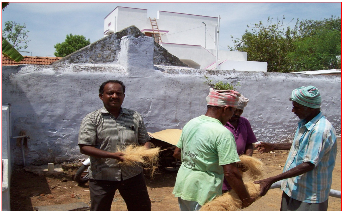
Plate 3.6 Wrapping coconut coir on corrugated flexible perforated PVC pipes (Gwalior)
