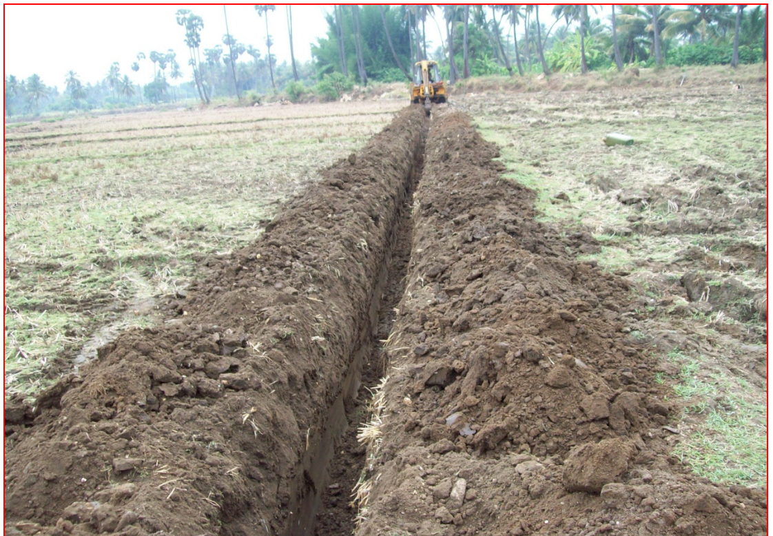
Plate 3.4 Trench making to required depth with JCB (15.014.2012)
