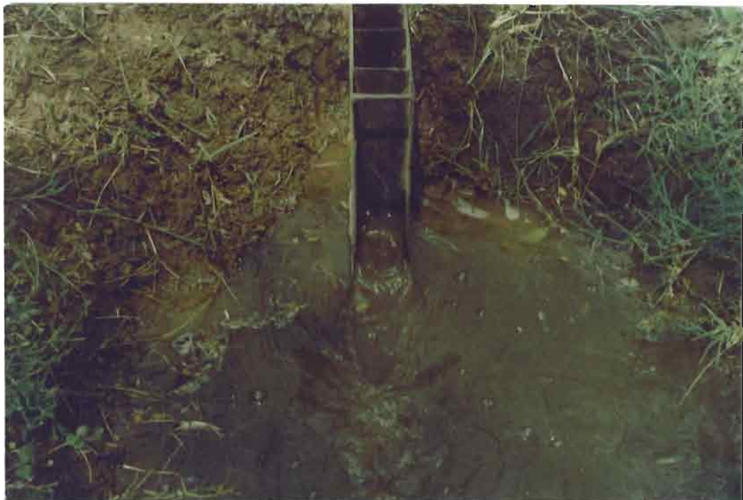
Plate No.5. Irrigation module installed in the field channel
