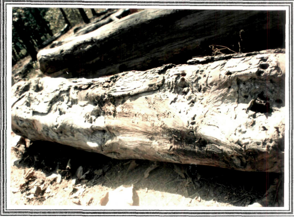
Plate 9: A teak log in a timber depot heavily ridden with borer holes.
