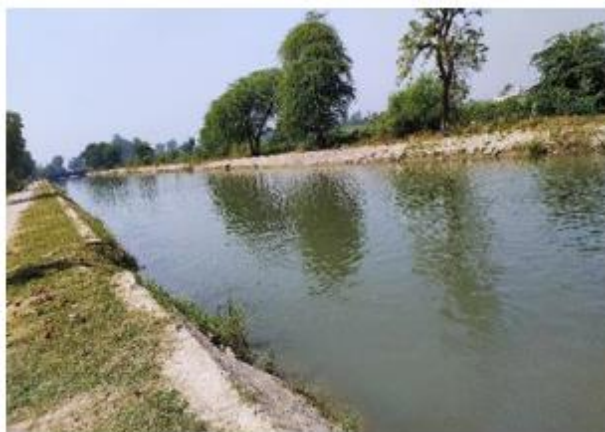
Plate 17: Water canal (near Satrod)
