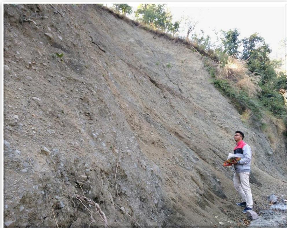
Fig. 3.6 Site View of Salri
