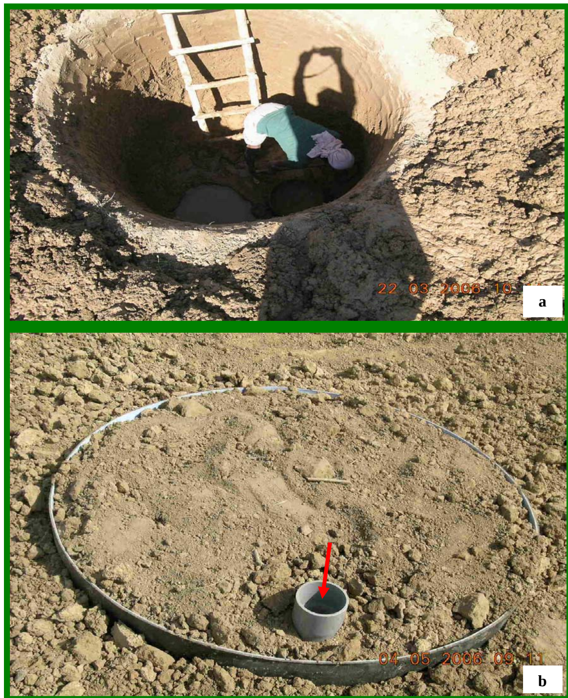
Fig. 3.2: (a) A cylindrical pit being dug for the fixation of lysimeter drum at the lysimeter site. (b) A freshly installed lysimeter filled up with field soil. Note the circular rim of the drum projecting above the soil. Arrow points towards the observation well installed in the lysimeter.
