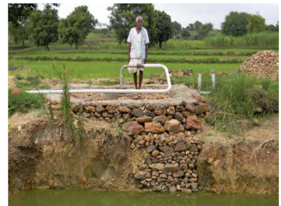
Rainwater harvesting through direct bore well recharge
