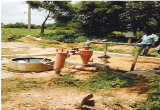
Bore well recharge structure for functional agriculture wells
