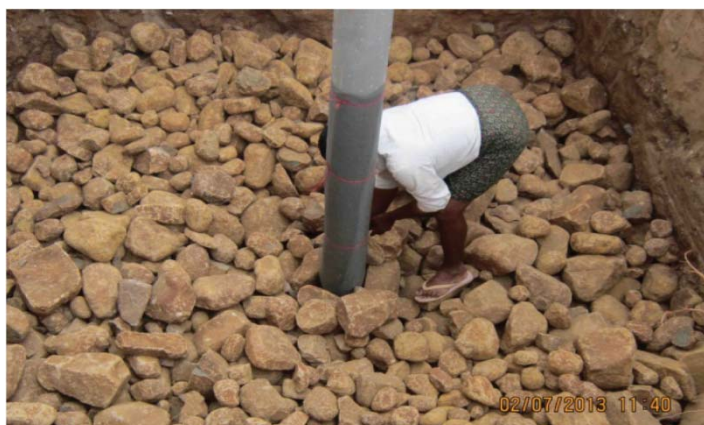
Renovated bund of a Small holes made on the casing pipe to allow rainwater to enter the bore well Water
