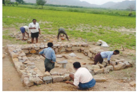
Construction of a recharge structure around existing bore well
