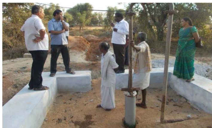
A pit around the existing bore well is filled with filter material
