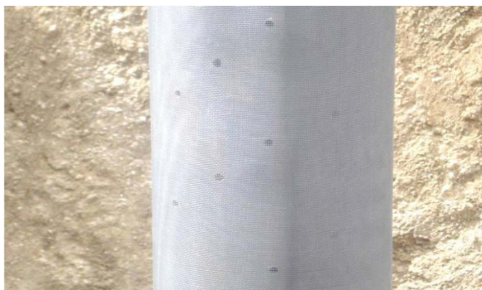
Renovated bund of a Small holes made on the casing pipe to allow rainwater to enter the bore well Water
