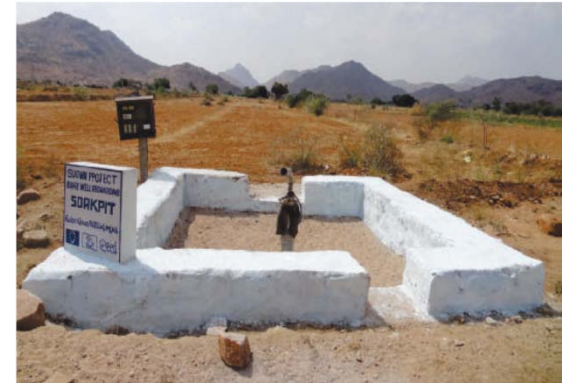
Bore well recharge structure for functional agriculture wells
