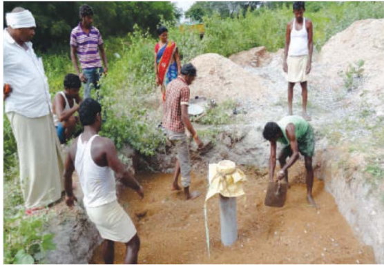
Construction of a recharge structure around existing bore well
