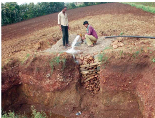
Rainwater harvesting through direct bore well recharge
