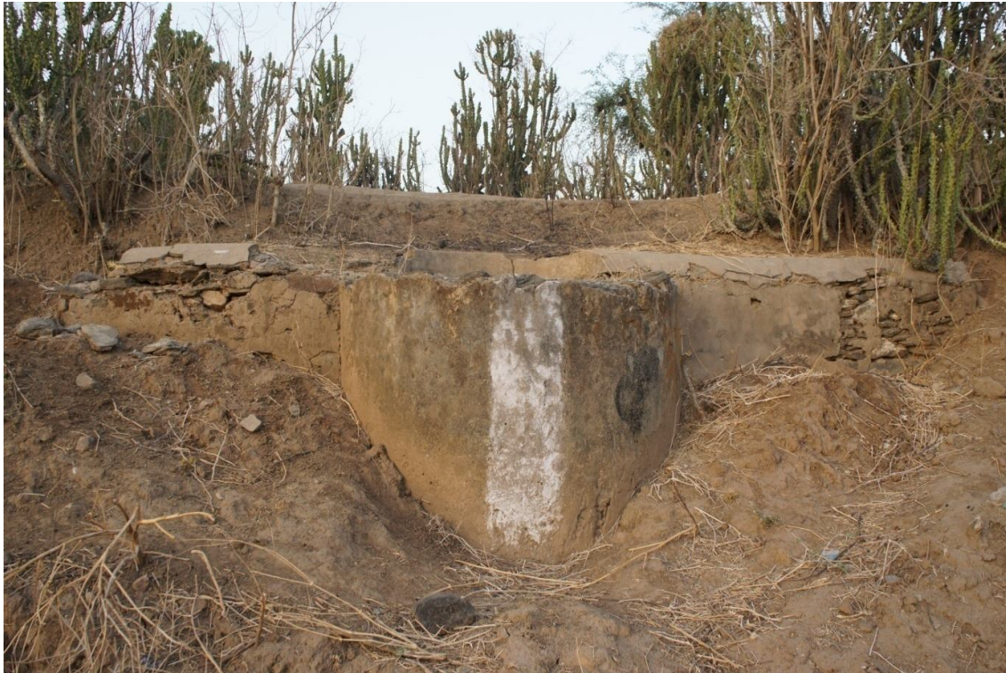
Plate 3.8: Sluice at Baran Nadi
