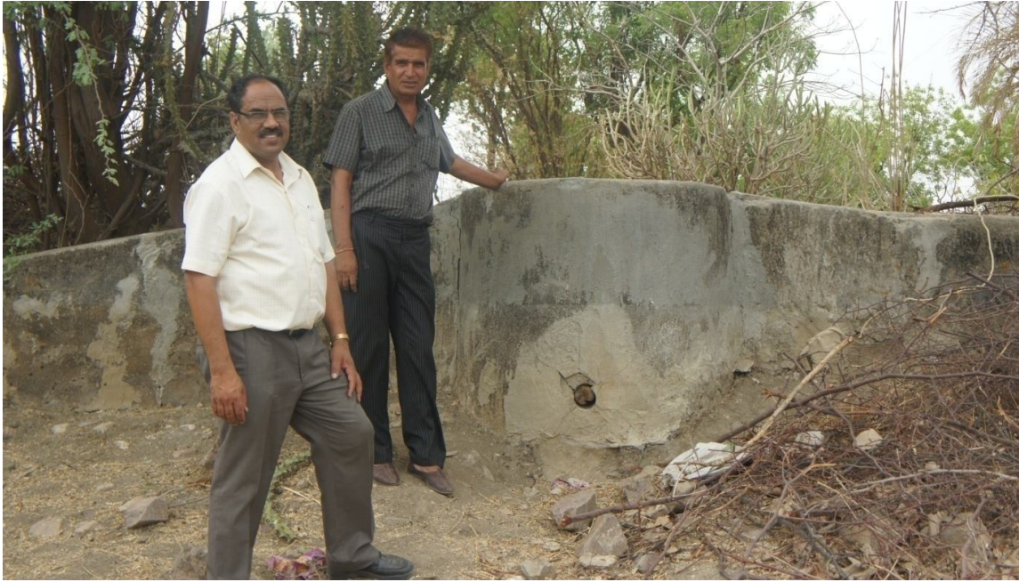
Plate 3.4: Sluice at Chalaniya Nadi
