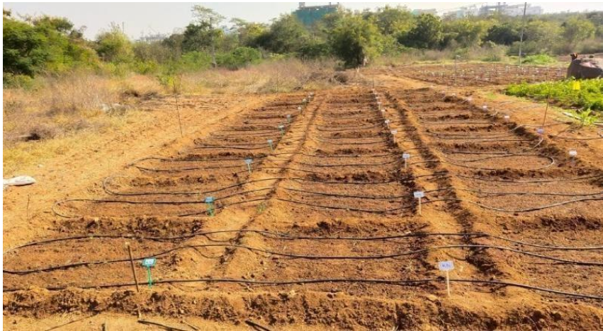
After Installation of drip
