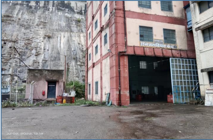
Plate 10. Hydeo-electricity power generation Unit Dimbhe
