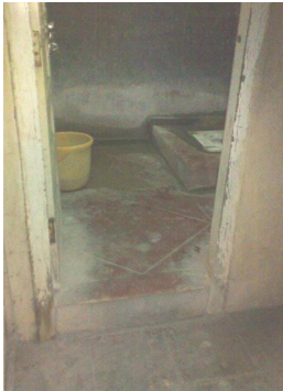
Access to bathroom
