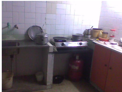
Kitchen work counters
