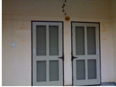
Double shuttered Entrance Doors
