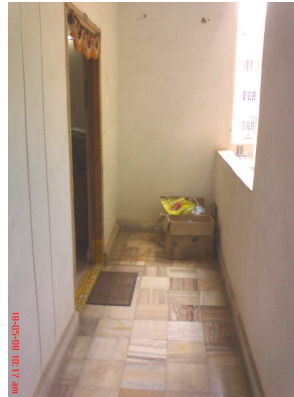
Entrance door with threshold
