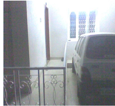
Entrance with ramp and parking
