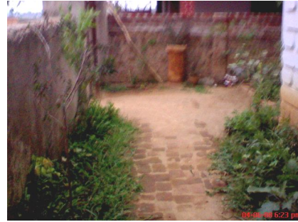
Uneven walk way within compound
