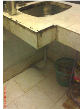
Knee space under sink in kitchen
