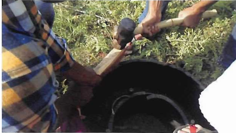
Plate 3.4. Installation of outer ring
