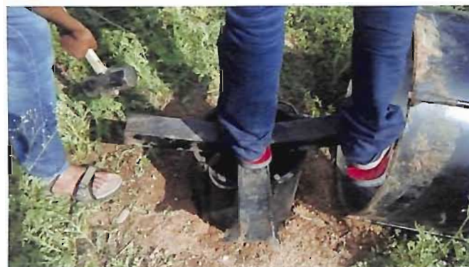
Plate 3.3. Installation of inner ring
