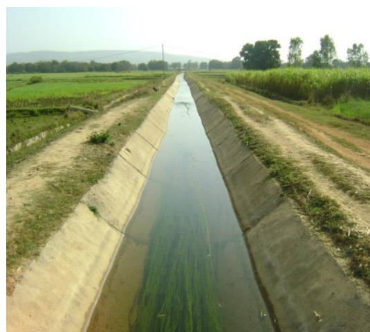
Plate 3.2 Main Canal of Govindgarh WUA
