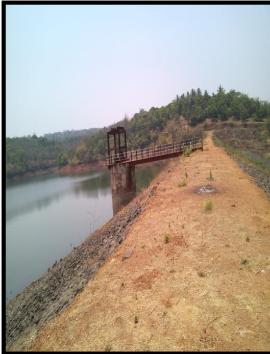
Fig.4.5 Outlet well (control gate)
