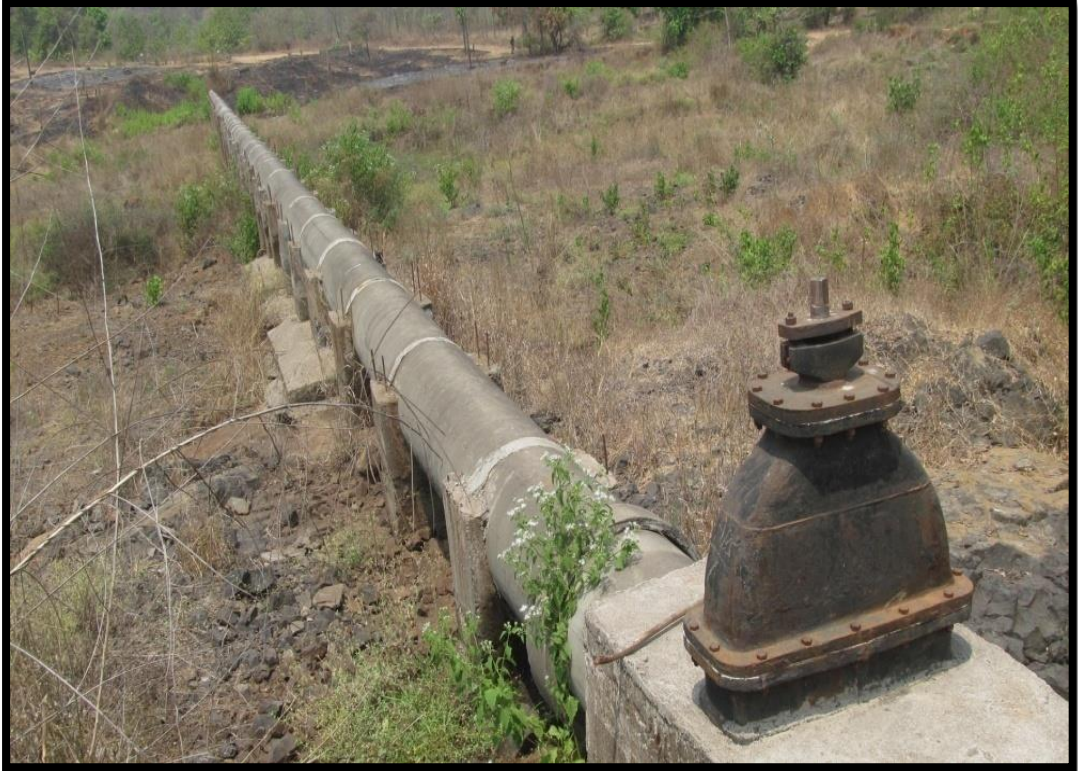
Fig.4.7 RCC mainline of LBC
