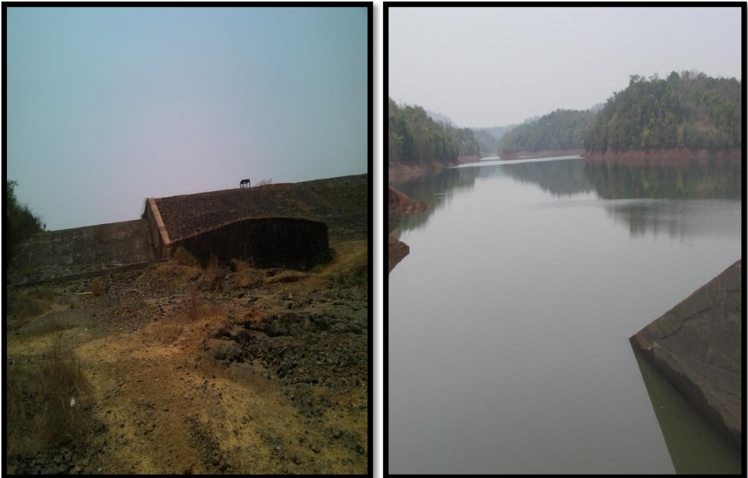
Fig 4.8 Earthen dam wall and water storage in the reservoir
