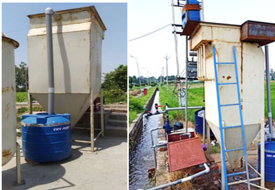
Fig. 4.2: Inclined Tube Clarifier Installation
