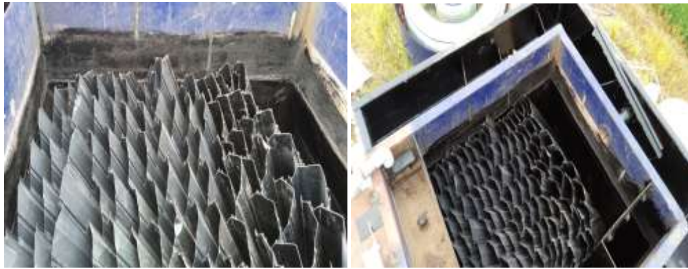
Fig. 4.1: Fabrication of Inclined Tubes Clarifier
