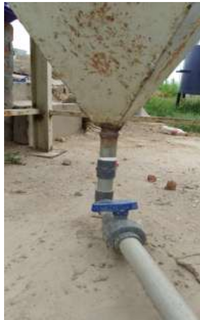
Fig. 4.5 Desludging valve
