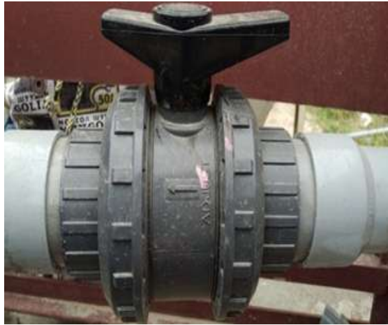
Fig. 3.1: Flow rate control valve
