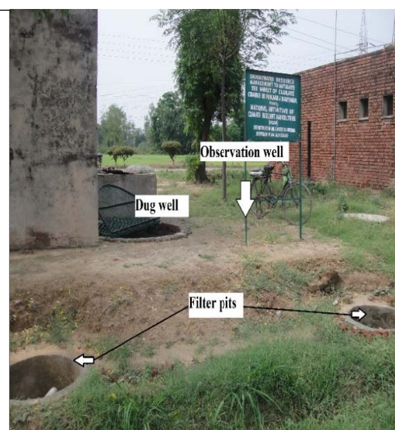
Fig. 3.6 View of abandoned well at site 2 and its dimensions
