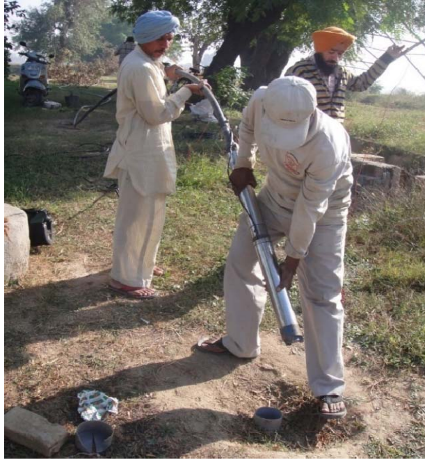
Fig. 3.10 Development of observation well
