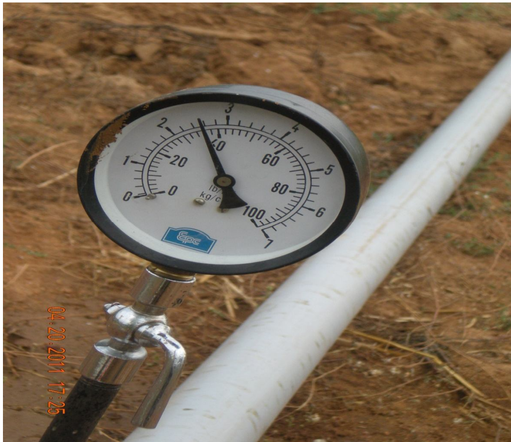
Plate 4.2.a. Measurement of pressure using pressure gauge on main line
