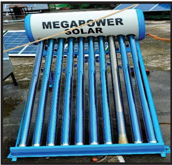
(c) Solar water heater
