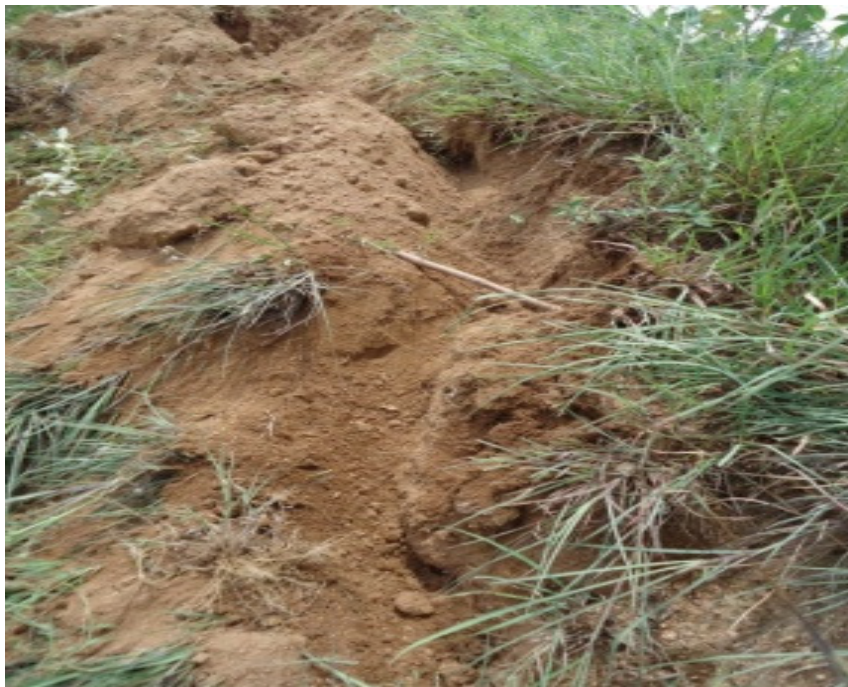
Plate 9. Excavated burrow on the bund
