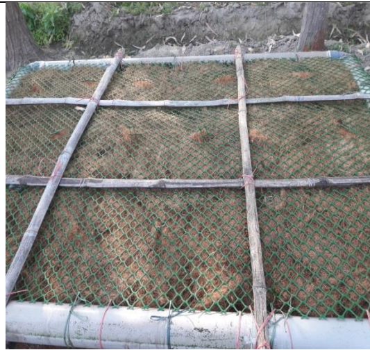
Step II- Binding with mess & bamboo
