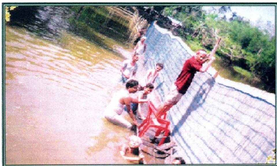
Figure 16. Researcher with the beel users during pen installation
