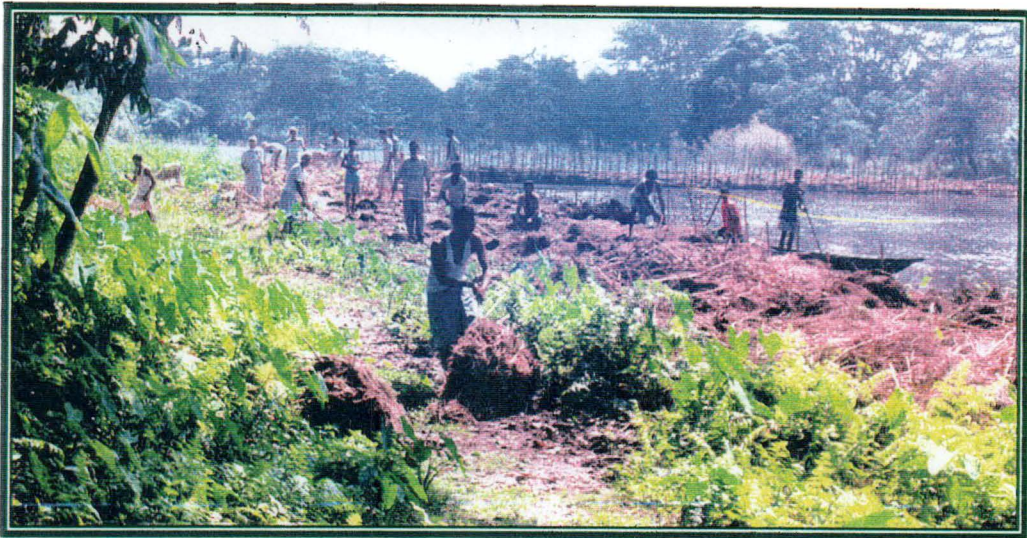
Figure 8 . Community members are renovating the Dek Beel .
