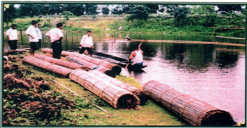
Figure 14. Split-bamboo screens with net are now ready for installation.
