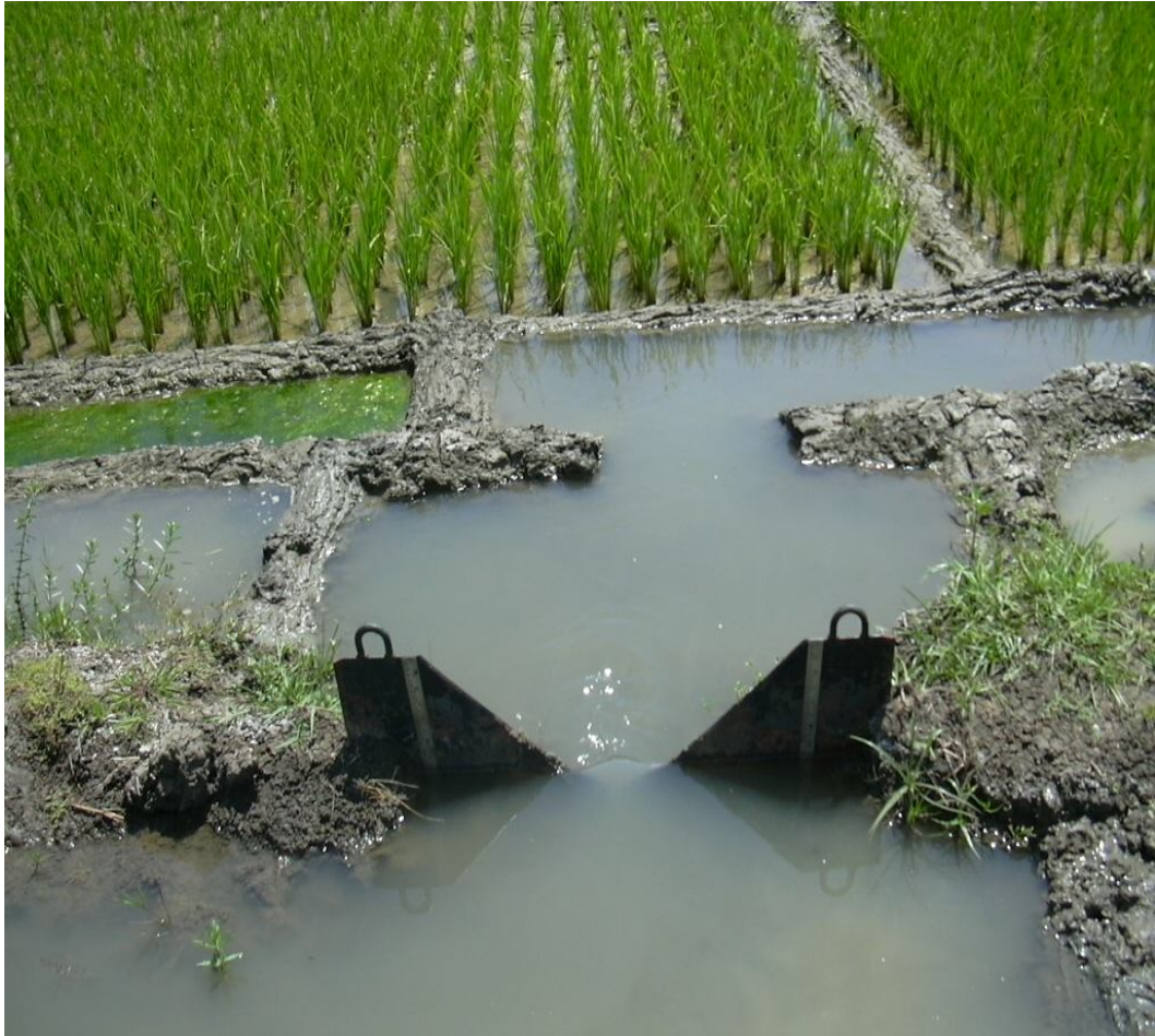
Plate 2: V-notch weir for measuring irrigation water
