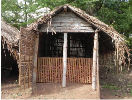
(T 1 ) Bamboo battens thatched roof structure without bottom ventilation (outside and inside view)
