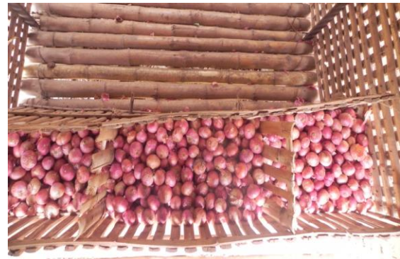
(T 3 ) Bamboo battens storage structure with AC sheet roofing with bottom and side ventilation (outside and inside view)
