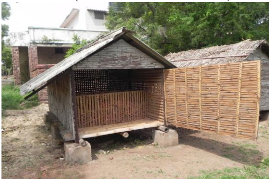
(T 3 ) Bamboo battens storage structure with AC sheet roofing with bottom and side ventilation (outside and inside view)
