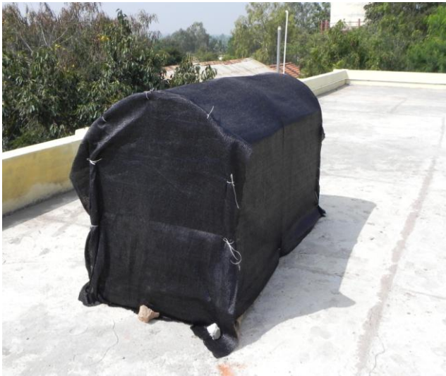
Curing under 35 per cent shade (outer view)
