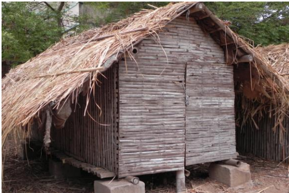
(T 2 ) Bamboo battens low cost storage structure with typha roofing with bottom and side ventilation (outside and inside view)
