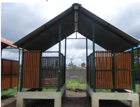
(T 4 ) Wooden battens storage structure with AC Sheet roofing and with bottom and side ventilation (outside and inside view)
