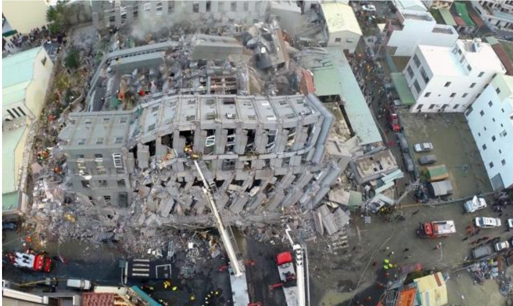
Fig.1.6 A Site where Buildings Collapsed is Seen in this Aerial Picture taken after a Powerful Earthquake Hit Tainan, Southern Taiwan, February 6, 2016.
