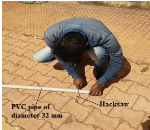
Plate 3.32 Cutting the pipes for device assembly
