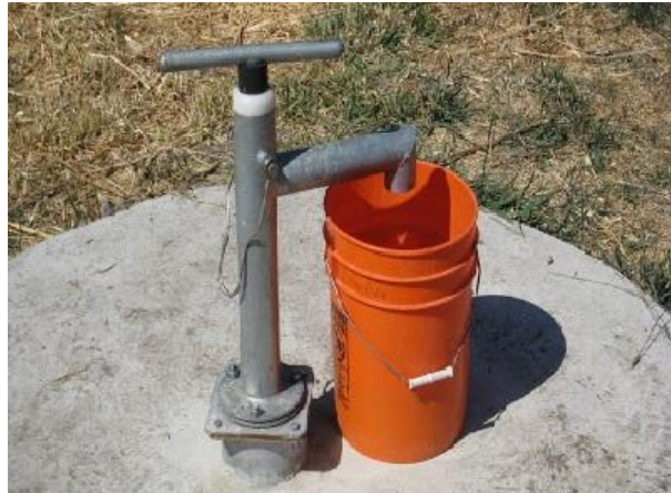
Plate 3.7 Direct Action Handpump
