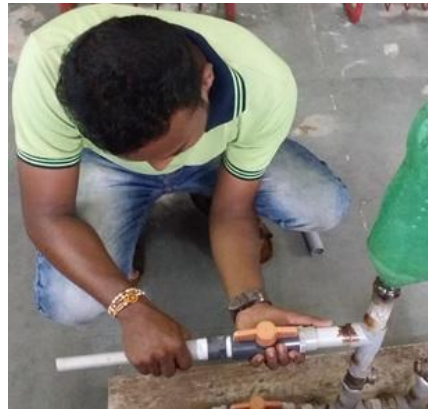
Plate 4.6 Fitting of control valve
