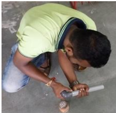
Plate 4.3 Fixing of elbow
