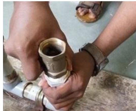
Plate 4.4 Installation of the waste valve
