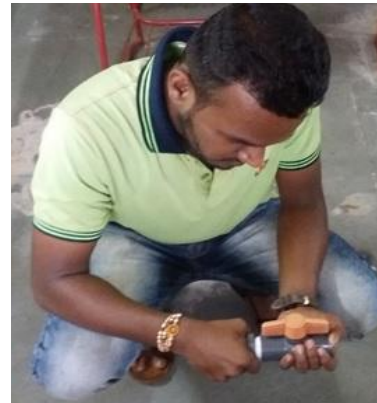
Plate 4.2 Use of Teflon tape around the MTA and joining control valve to neat fitting
