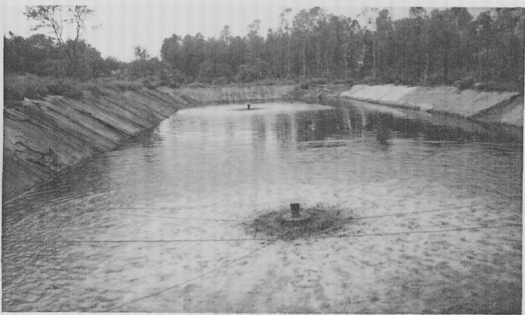
7. Aeration tank in Doon Valley distillery
