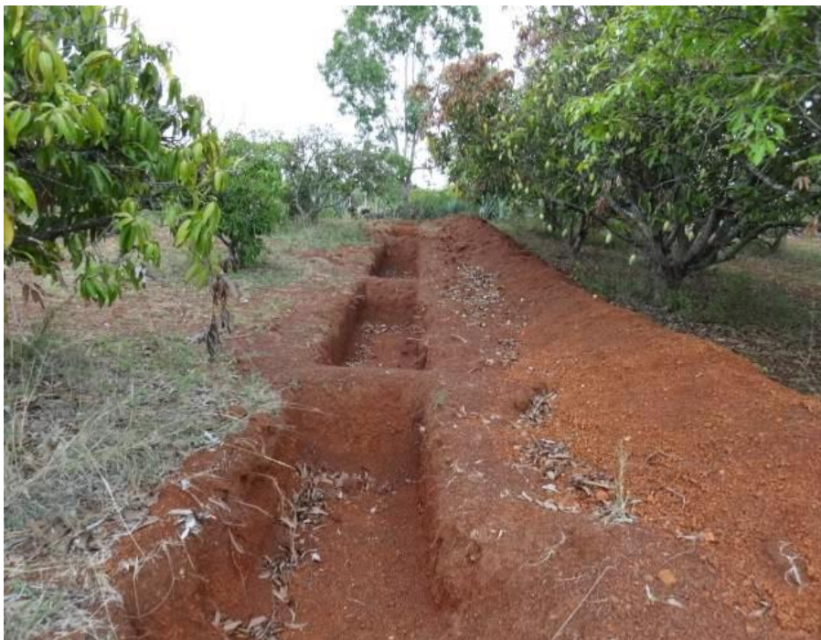
Plate 4.4: Trench cum bund constructed under PMKSY-WD in the study area
