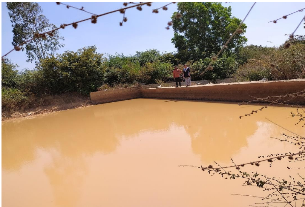
Plate 4.2: Check dam constructed under PMKSY-WD in the study area
