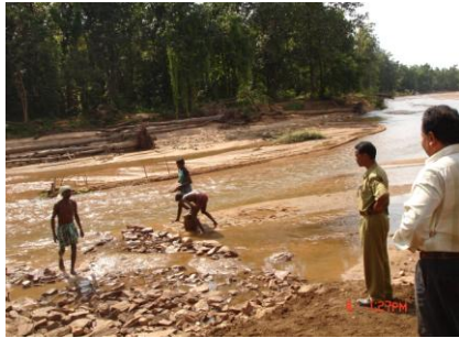
Construction of a rapta (road).
