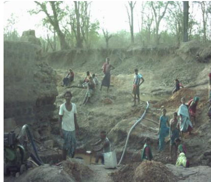
Construction of a stop dam.
