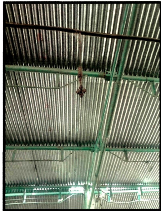
Plate VIII: Fogger provided to reduce heat stress at dairy farm of Kaushal Patel
