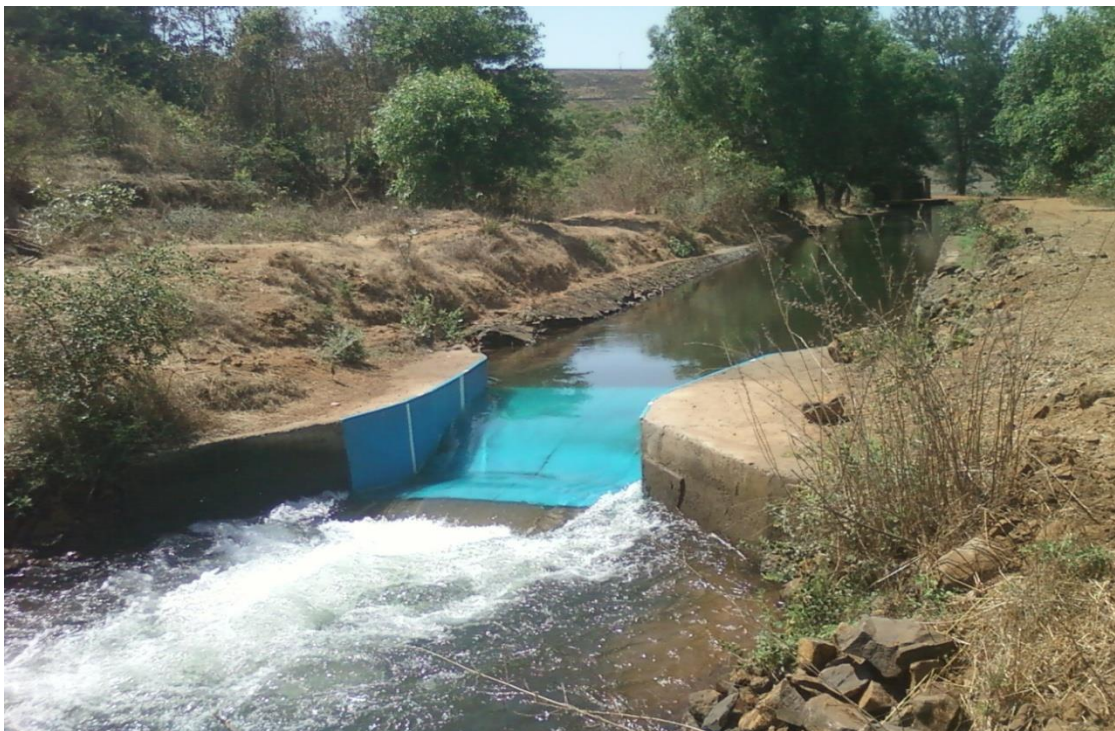
Plate No. 5 Flow measurement using Parshall flume on right bank canal
