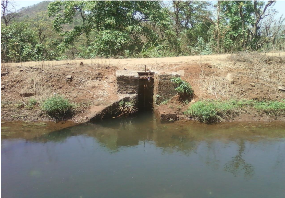
Plate No. 6 Gated outlets on right bank canal
