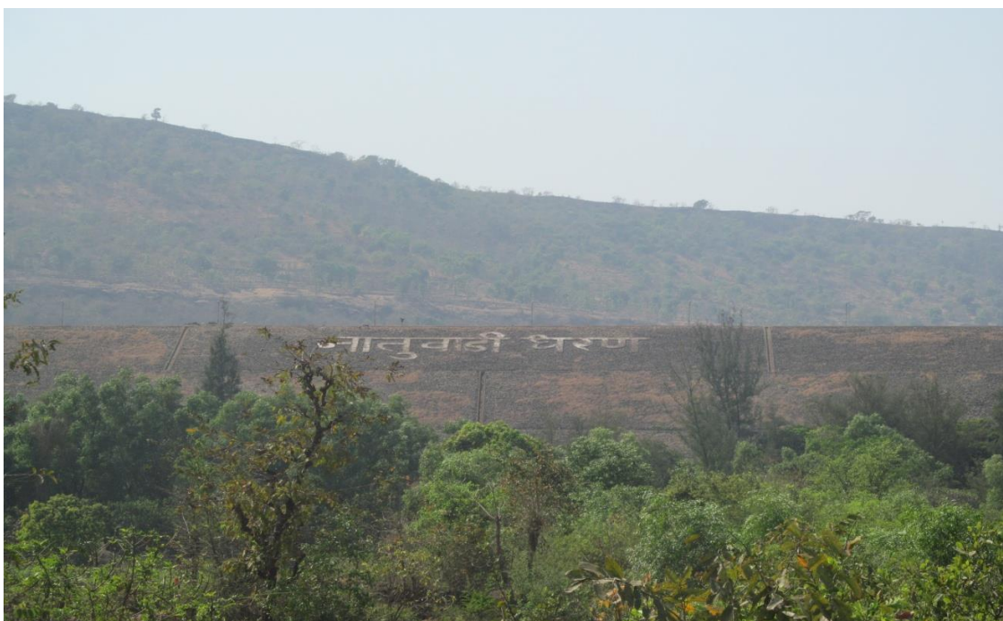
Plate No. 3 General view of Natuwadi medium irrigation project, Khed
