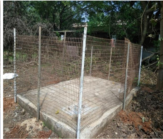
Fig. 8: Prepared compost bin
