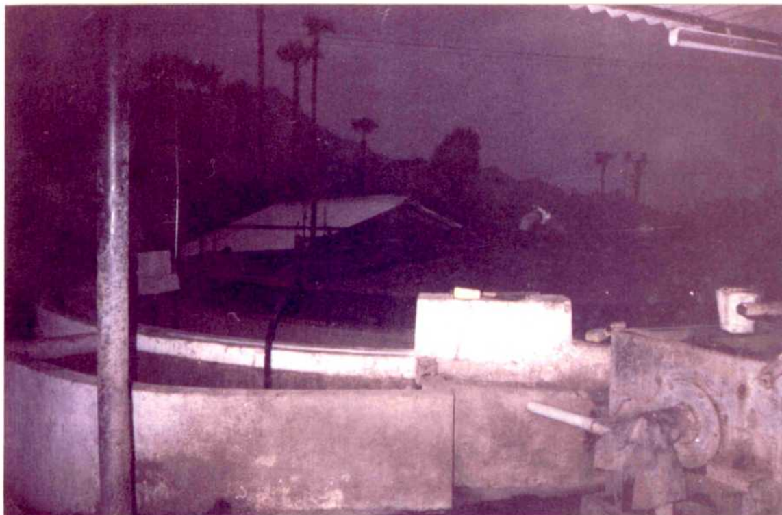
Plate No. 3.5 85 m 3 KVIC model biogas plant
