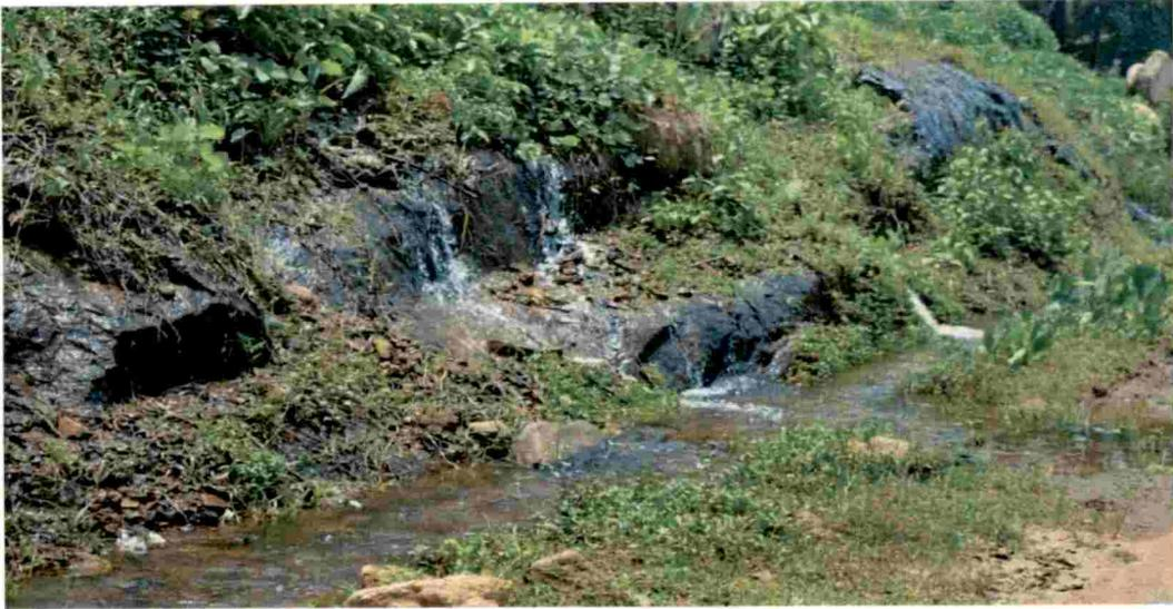
**Figure 26. Leakage from main canal**
