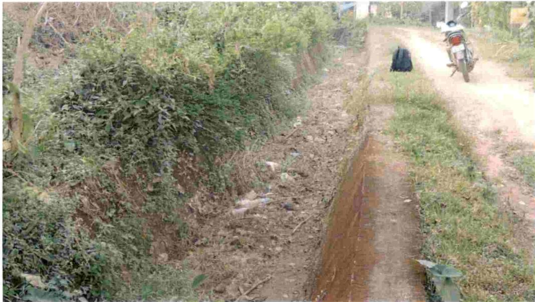
**Figure 28. Improper maintenance of branch canals**
