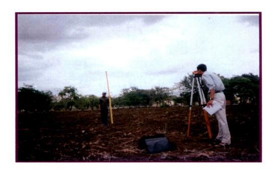
Plate 1 Grid survey using dumpy level.
