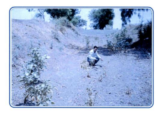
Plate No. 5. Measurement of silt deposition at cement check dam.
