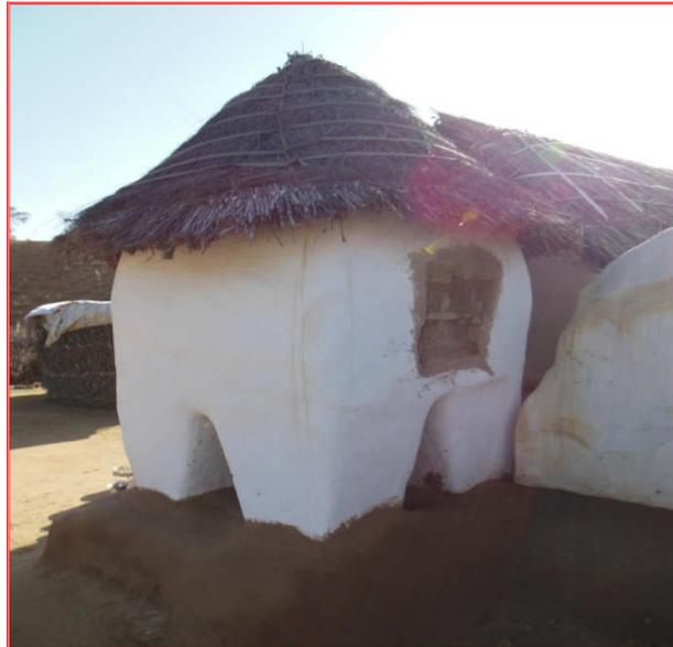
Photo 5 : *Kothi* – the grain storage structure
